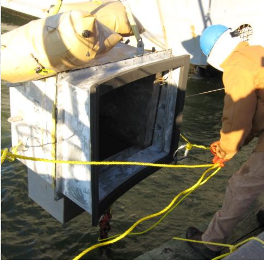
Dry Chamber Ready for Installation
