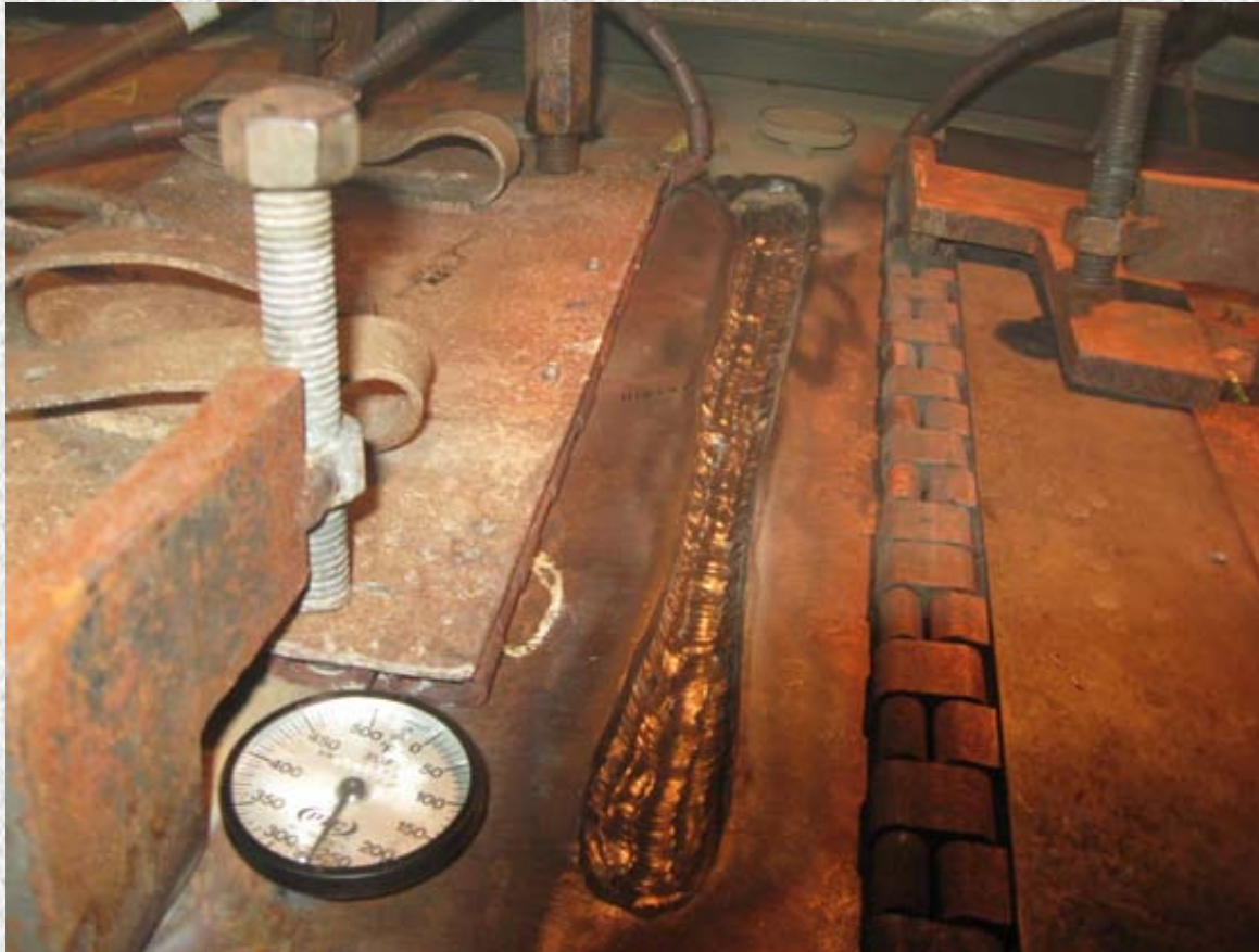
Dry Chamber Weld – Root Pass with Pre-Heat
