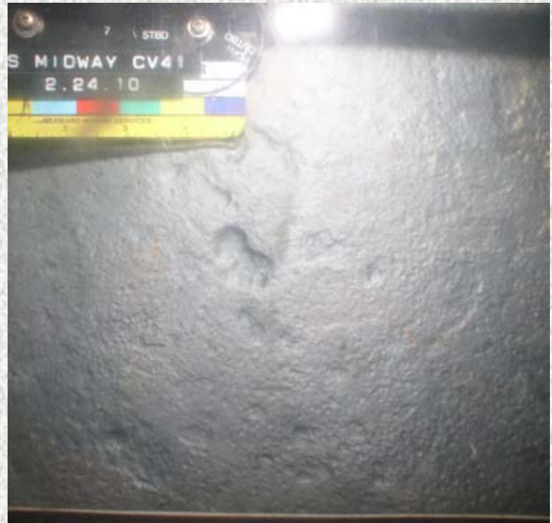
Area Prepared to Bare Metal for U/W Coating
