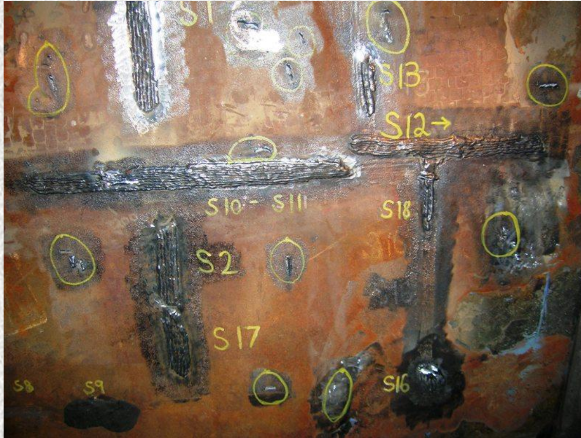
DDG Rudder Repair in a Dry Chamber
