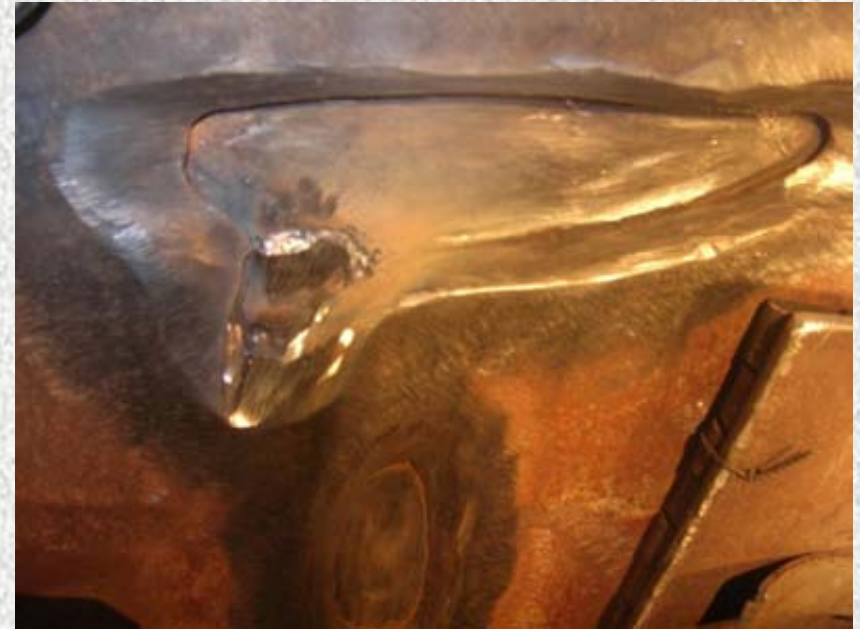
Weld Prep in Dry Chamber
