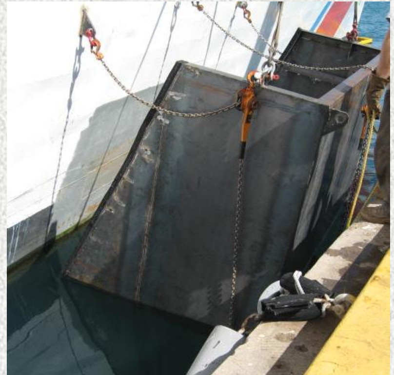
Rigged for Installation
