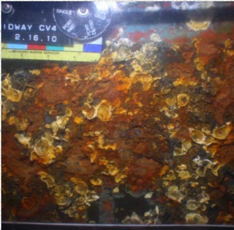
Heavy Fouling and Corrosion in Work Area
