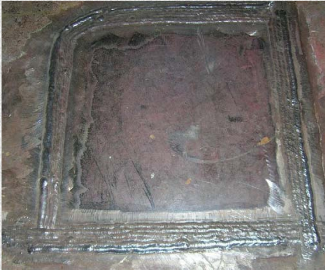
Completed Weld from Interior of Hull
